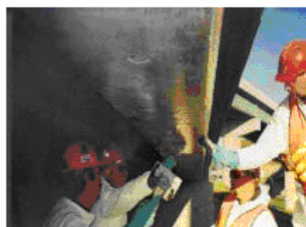
(c) Application of Putty
