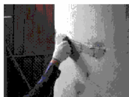
(a) Corrosion resistance treatment
