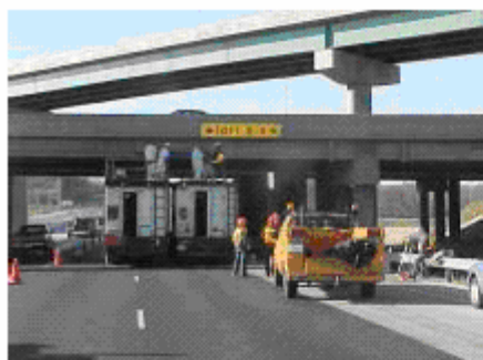
(a) Overall View
