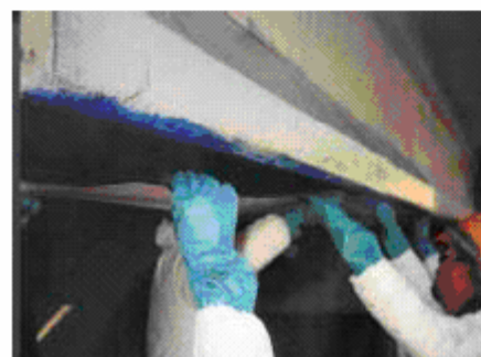
(e) Manual Lay-up of CFRP Sheet
