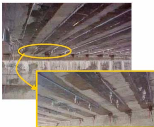
(b) Bolted CFRP Plates
